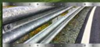
This type is commonly used on Toll Roads or highways that are passed by heavy vehicles or at high speed.
